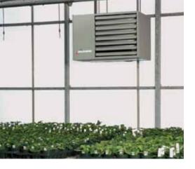
PTP unit heaters can have manual or automatic operation and use natural or propane gas.
