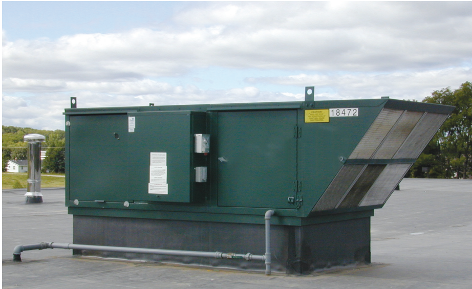
Direct gas-fired air heaters are a cost effective means for delivering clean, tempered ventilation air to purge contaminants from a building or provide clean, tempered outdoor air for odor control.
